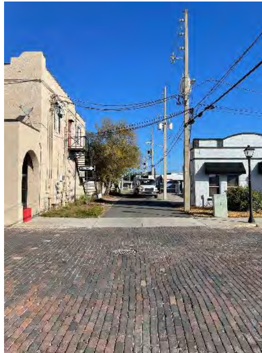
Existing alley conditions
