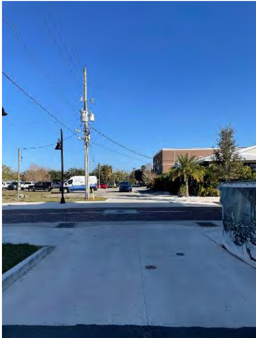
Existing alley conditions
