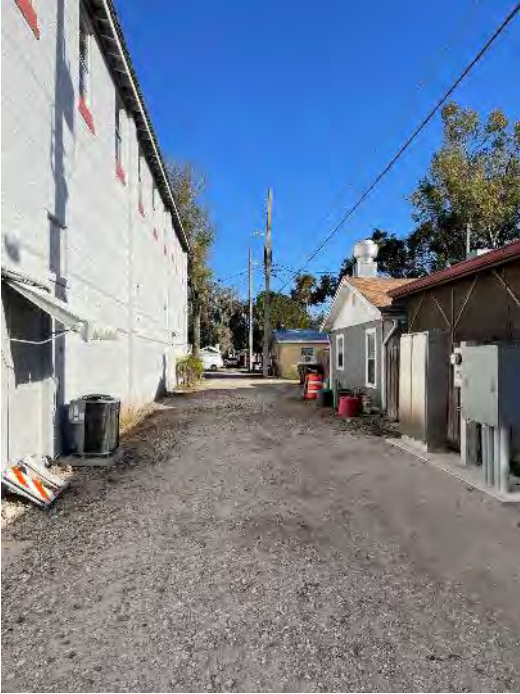
Existing alley conditions
