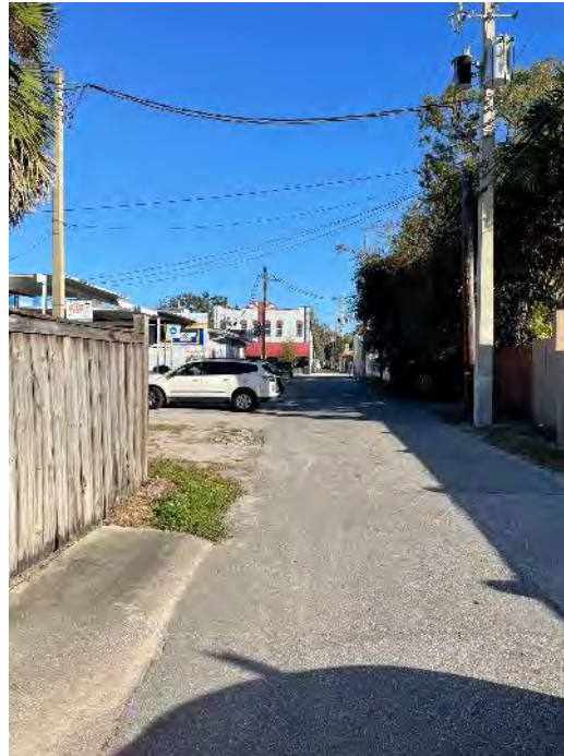
Existing alley conditions
