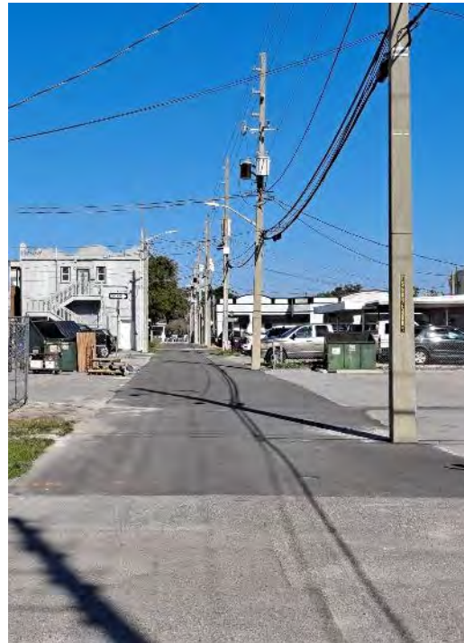
Existing alley conditions
