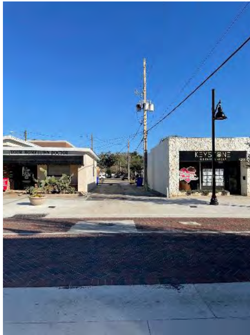
Existing alley conditions
