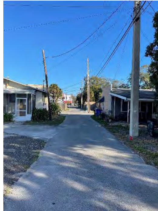
Existing alley conditions
