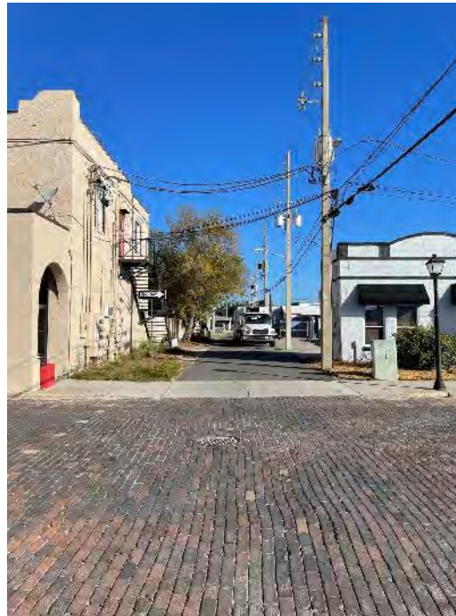
Existing alley conditions
