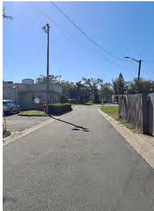
Existing alley conditions
