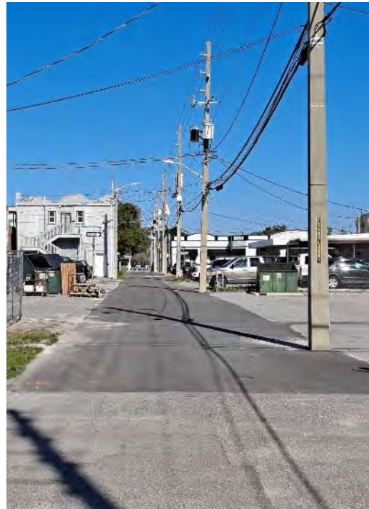
Existing alley conditions
