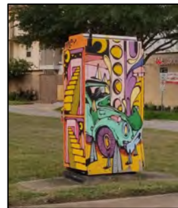
Painted utility box
