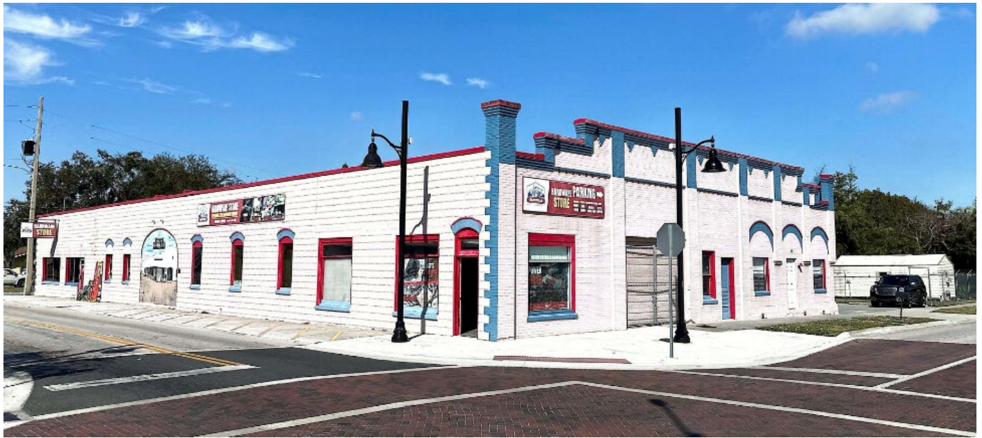
Figure 2 – 1410 10 th Street (East and South Elevations)
